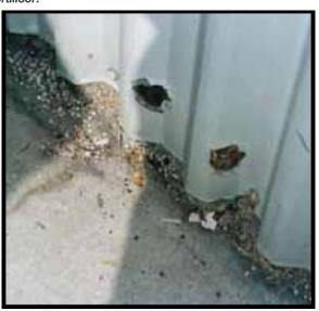
Figure 2: Build-up on a purlin.
