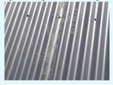
Figure 2: Roofing with sunscreen damage
