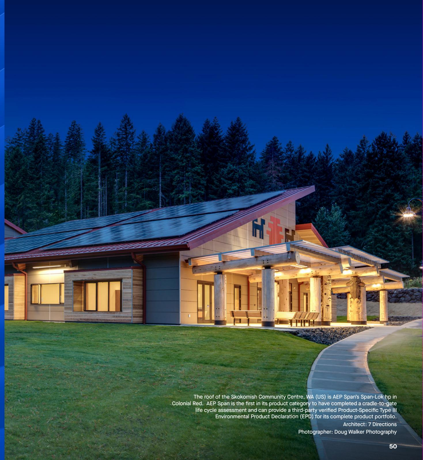
The roof of the Skokomish Community Centre, WA (US) is AEP Span's Span-Lok hp in Colonial Red. AEP Span is the first in its product category to have completed a cradle-to-gate life cycle assessment and can provide a third-party verified Product-Specific Type III Environmental Product Declaration (EPD) for its complete product portfolio.
