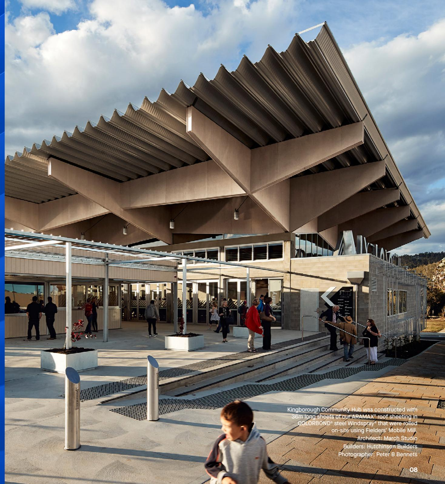
Kingborough Community Hub was constructed with 36m long sheets of our ARAMAX® roof sheeting in COLORBOND® steel Windspray® that were rolled on-site using Fielders' Mobile Mill.
